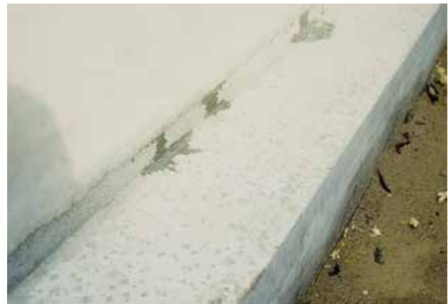
Simple injection process on site
