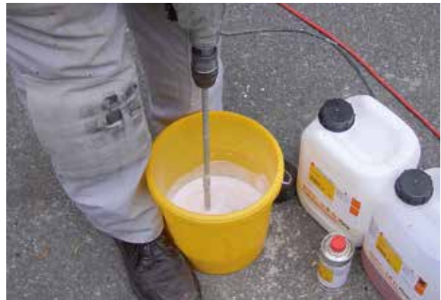
Mixing of an acrylic based Sika injection resin
