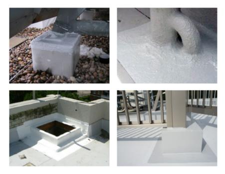
Sikalastic®-621 LIQUID APPLIED MEMBRANE IS THE SOLUTION FOR DIFFICULT DE-TAILS OF A SINGLE PLY MEMBRANE ROOFING SYSTEM, BECAUSE OF ITS VERSA-TILITY AND TIME SAVING INSTALLATION.
