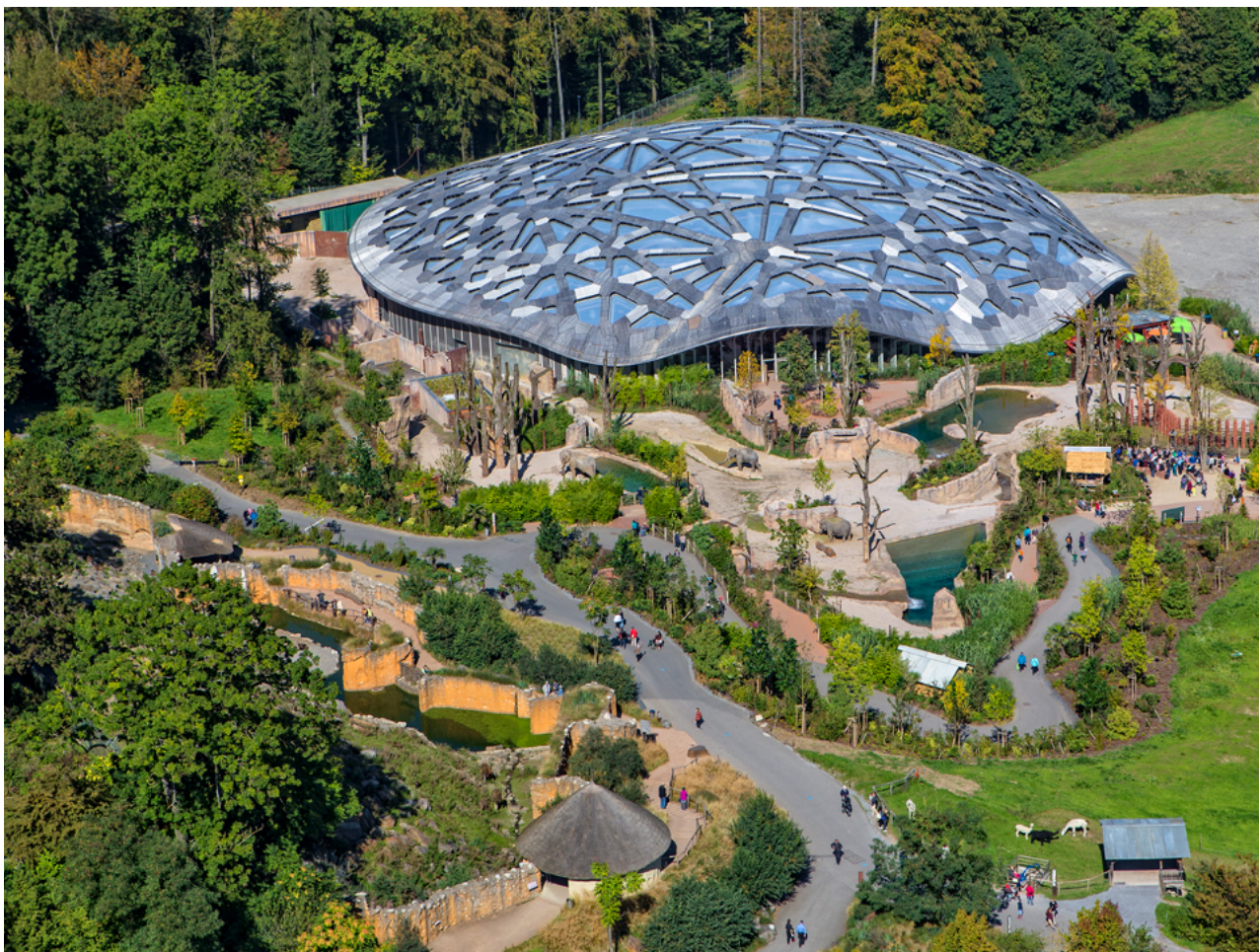
A sustainable roofing solution from Sika was installed in the elephant enclosure in Zurich Zoo.
