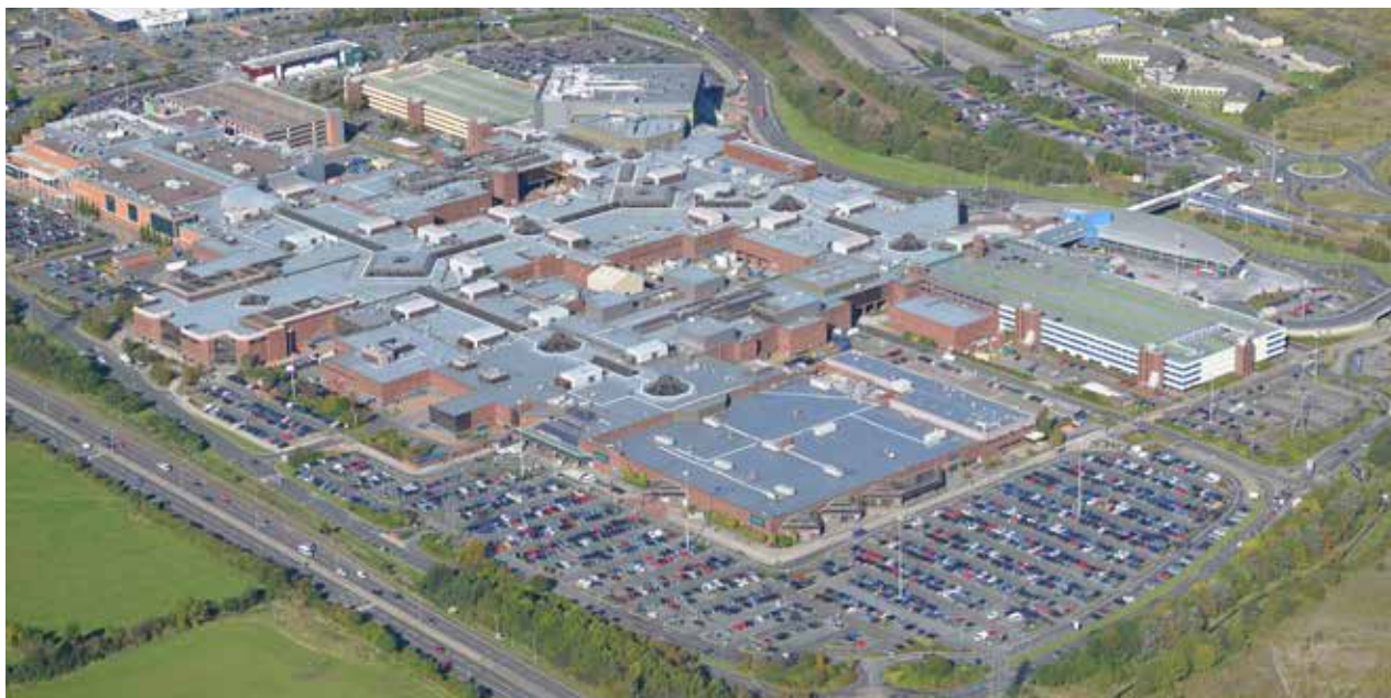
Shopping center MetroCentre (20,000 m 2 ), Gateshead, UK.
