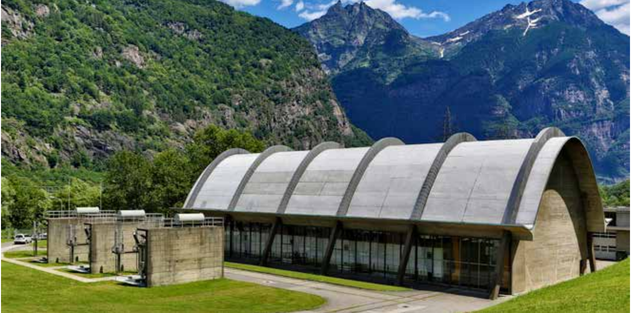
Hydroelectric power plant in Personico, Switzerland.
