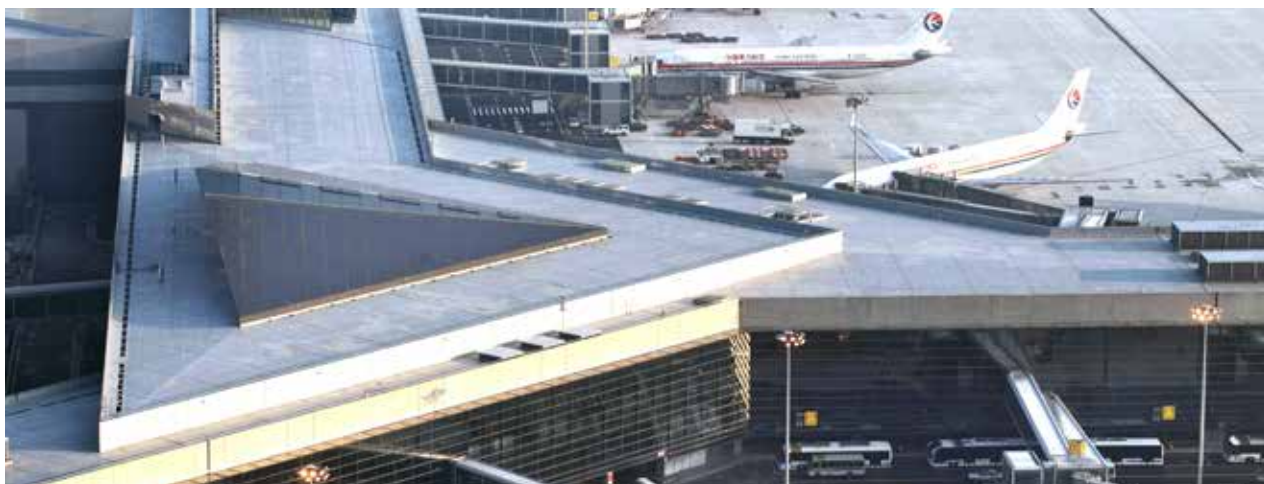
Shanghai Hongqiao International Airport, China.
