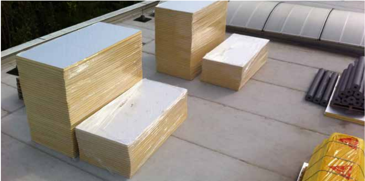
Roofing of Reál Shop, Dunajváros, Hungary.
