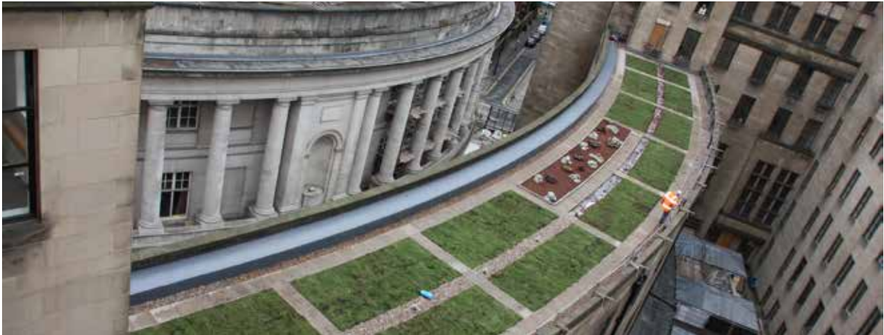
Green roof on Manchester Town Hall, UK.
