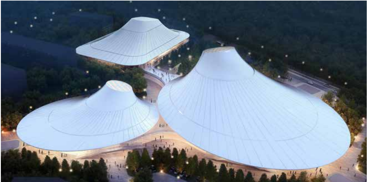
Indoor Stadium of Yulin Vocational and Technical College, China.
