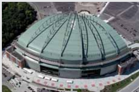
Miller Park, Milwaukee, USA
