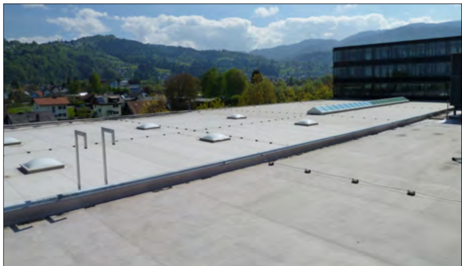
Fig. 3: Overall view of the roof of the Meusburger Building in Wolfurt (Austria)
