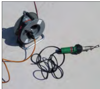
Fig. 6: Hot air welding of new to existing membranes ( Sarnafil® TS 77-18 ) Meusburger Building in Wolfurt (Austria)
