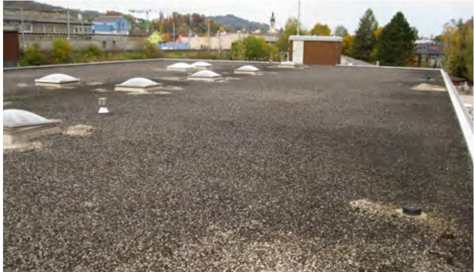
Fig. 4: Overall view of the roof of the Brunner Building in Flawil (Switzerland)
