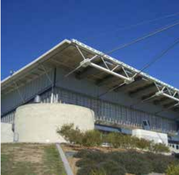
Project year: 1981 | Australian Institute of Sport AIS Arena Canberra, Australia
