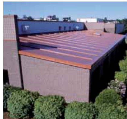
Special Roof Design
