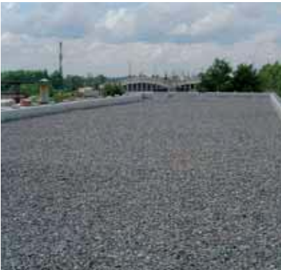
Gravel Ballasted Roofs
