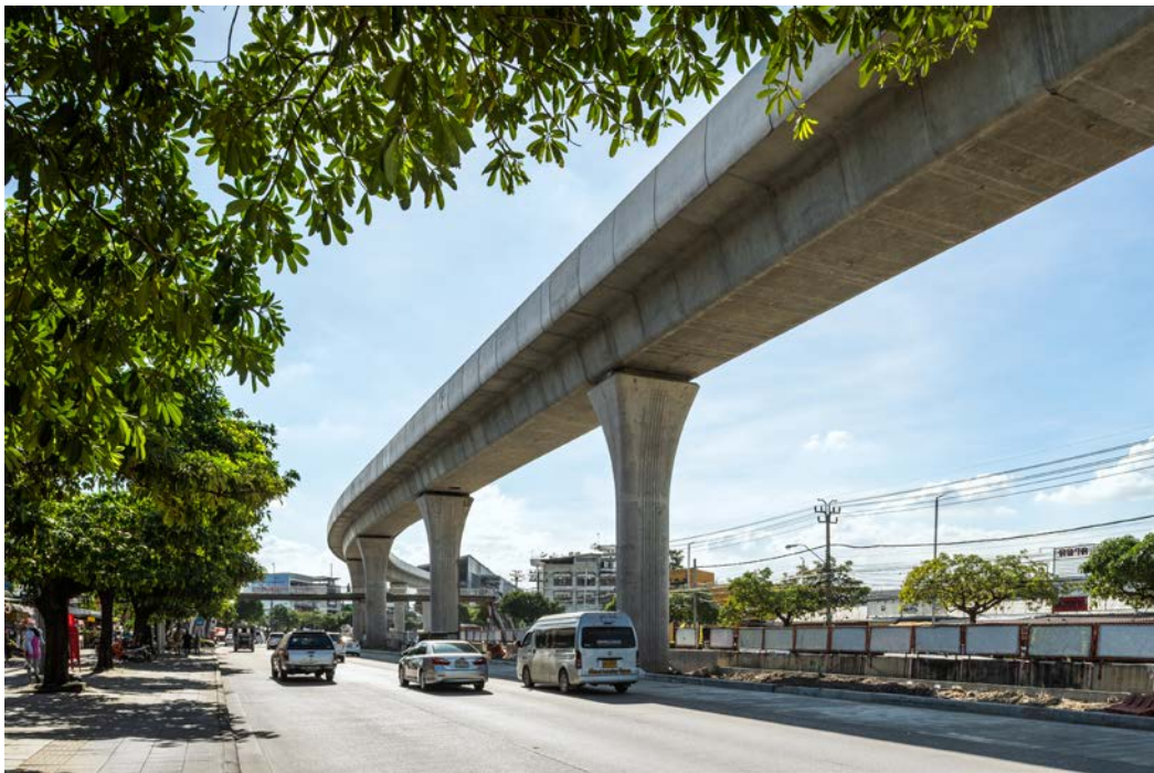
The MRT Orange Line consists of underground and overground rail systems. The comprehensive service delivered by Sika experts on site was invaluable for the project's success.
