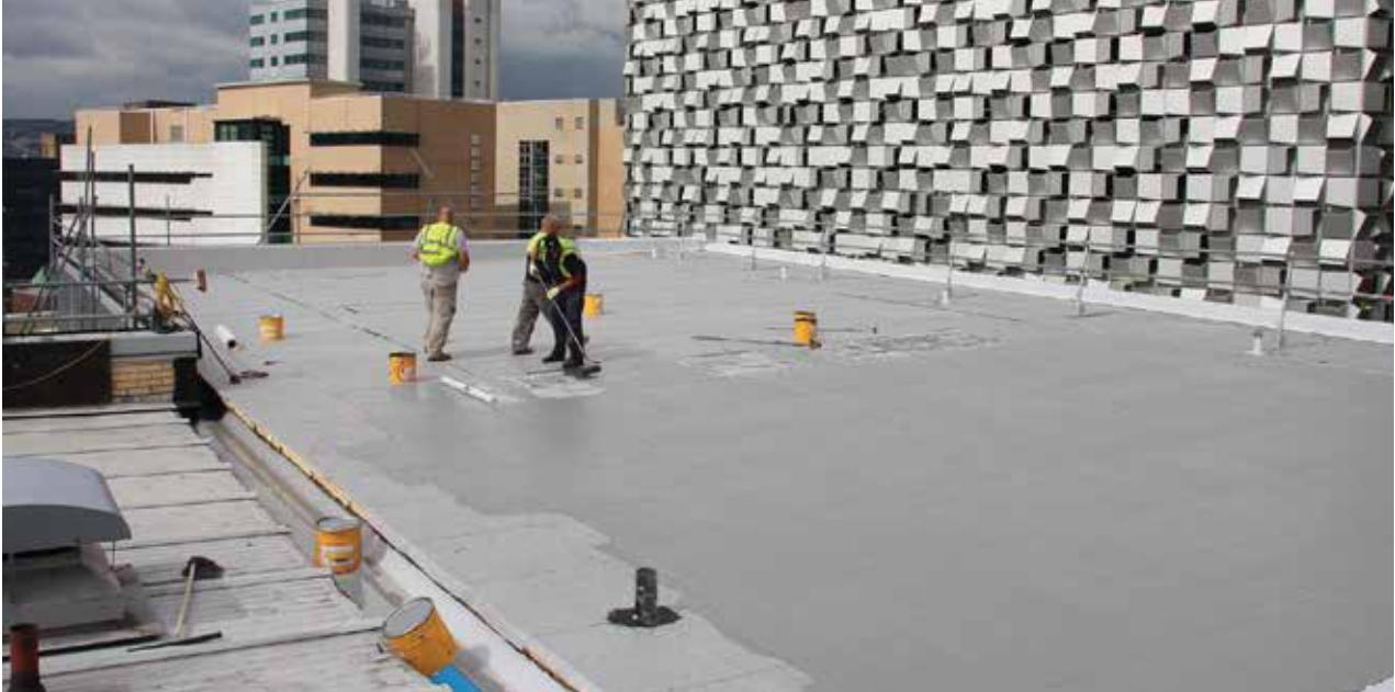
Liquid-applied membrane application, Hallam University, Sheffield, UK
