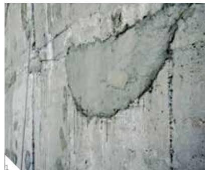
1 Hand applied Sika MonoTop® repair mortar. 2 Typical large damages to be repaired using dry spray technique.
