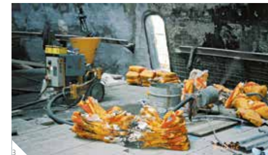
1 Internal application of Sika spray applied repair mortars in a cooling tower refurbishment. 2 Difficult shaped support structures easily repaired with SikaCem® Gunite 133. 3 Sika Aliva dry spray equipment in operation applying SikaCem® Gunite 133 inside a cooling tower.
