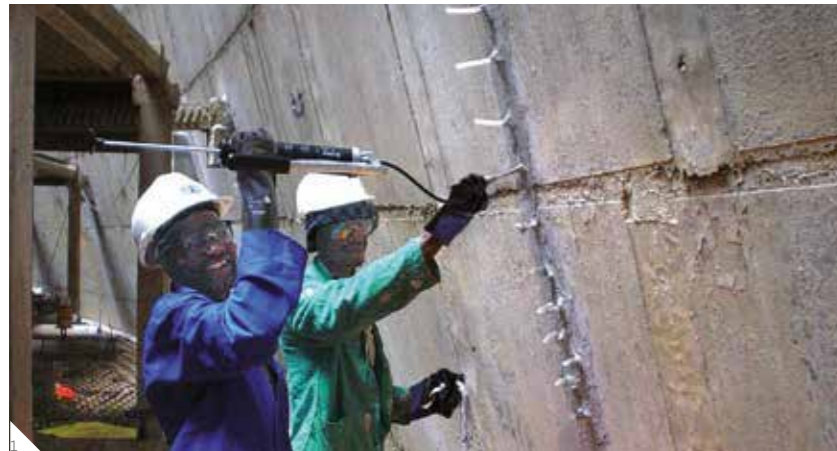
1 Structural bonding of cracks to restore structural integrity with Sika® Injection resin. 2 Crack-sealed with Sikaflex sealant and overcoated with Sikagard®-680 S protective coating.
