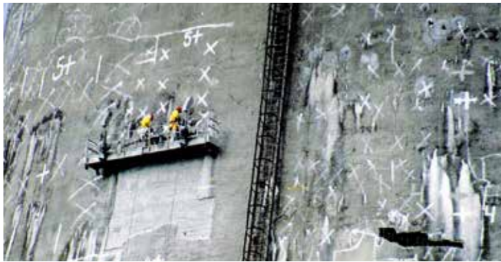
Break-out and removal of damaged concrete areas marked for repair in the condition survey.
