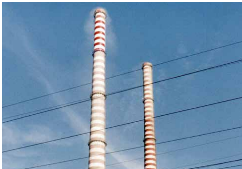
Chimneys in direct sunlight indicating variations in thermal exposure which are further exacerbated by the effects of the downward flow of hot exhaust gases during periods of temperature inversions.
