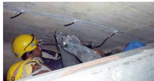
Crack Injection.
