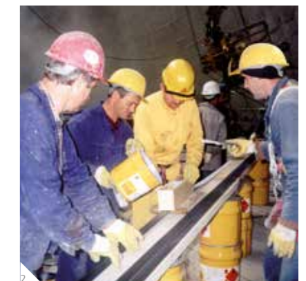
1 Sika CarboDur® CFRP plates being bonded with Sikadur® epoxy adhesive directly to the repaired external concrete surface at the top of a cooling tower for increased restraint. 2 Sikadur® adhesive application to the Sika CarboDur® plate. 3 Easy application of the Sika CarboDur® plates from powered access cradles.
