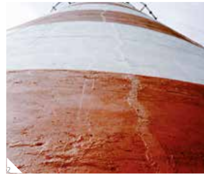
1 Structural bonding of cracks to restore structural integrity with Sika® Injection resin. 2 Crack-sealed with Sikaflex sealant and overcoated with Sikagard®-680 S protective coating.
