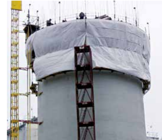
Sika Icosit®-2406 epoxy coating applied inside a cooling tower. Right: Slip-forming a new concrete chimney base structure with Sika® ViscoCrete® technology.
