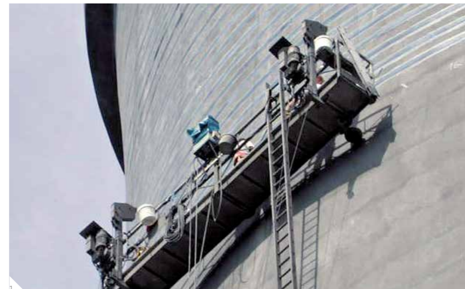
1 Sika CarboDur® CFRP plates being bonded with Sikadur® epoxy adhesive directly to the repaired external concrete surface at the top of a cooling tower for increased restraint. 2 Sikadur® adhesive application to the Sika CarboDur® plate. 3 Easy application of the Sika CarboDur® plates from powered access cradles.
