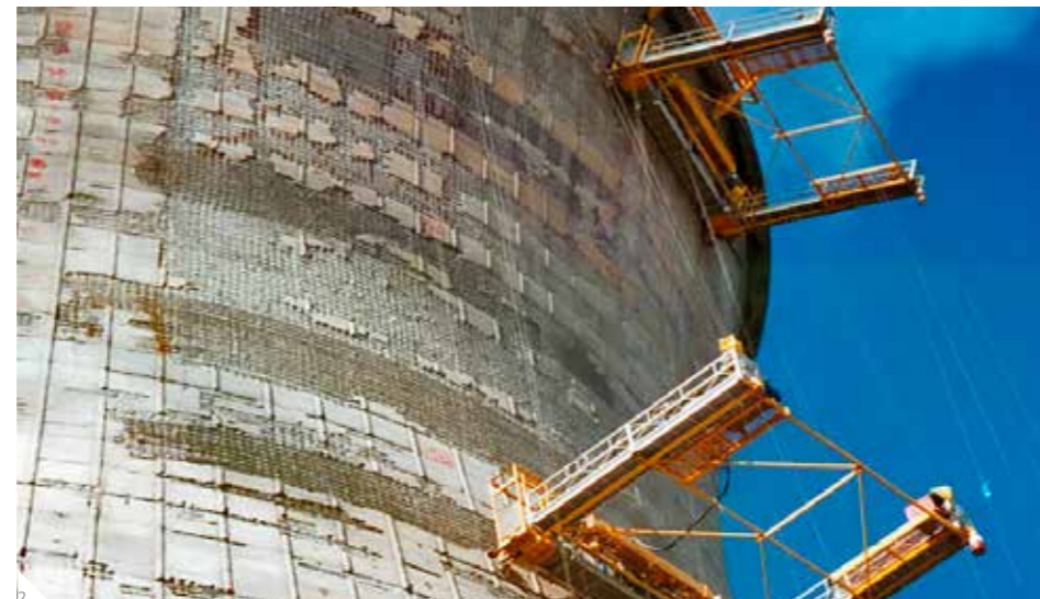
1 Hand applied Sika MonoTop® repair mortar. 2 Typical large damages to be repaired using dry spray technique.
