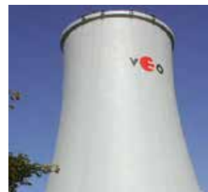
Autumn 2004, surface fully coated with Sikagard®-680 S concrete color.
