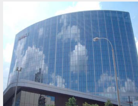
Hotel Hyatt Russia: Concrete refurbishment with various Sika Mortars
