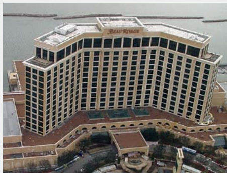
The MGM Beau Rivage USA: Sika roofing solution for the 29story high building
