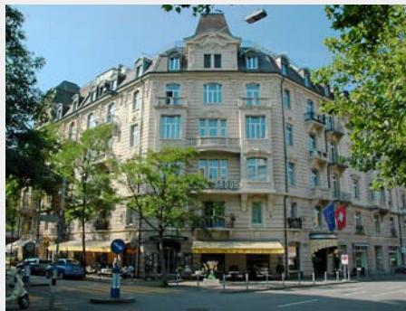
Hotel Ambassador Switzerland: Waterproofing and refurbishment solutions
