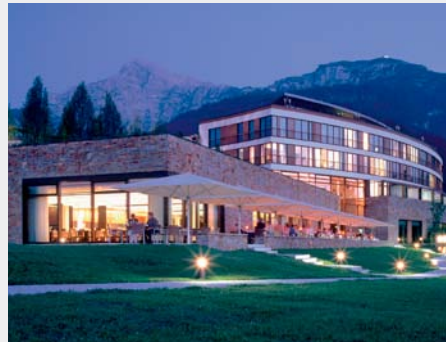
Resort Hotel Intercontinental Germany: Waterproofing with Sika floor lining for kitchenfloors
