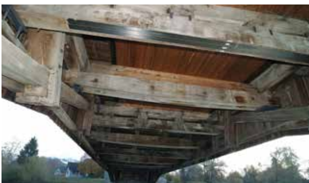
CarboDur® strengthened crossbeam
