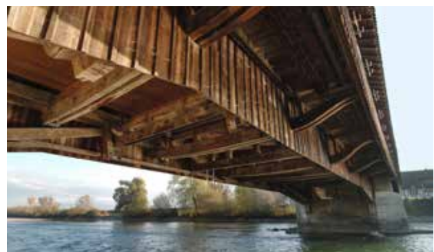
Bottom view of strengthening system
