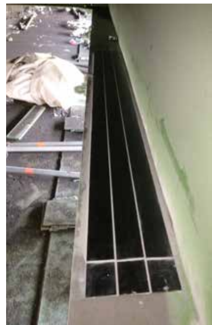
Two layers of Sika CarboDur®
