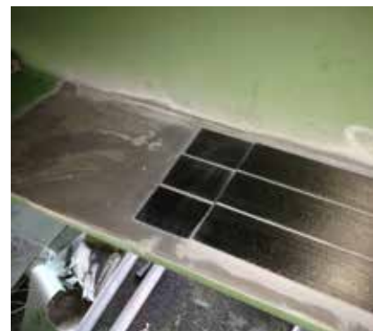
Two layers of Sika CarboDur®
