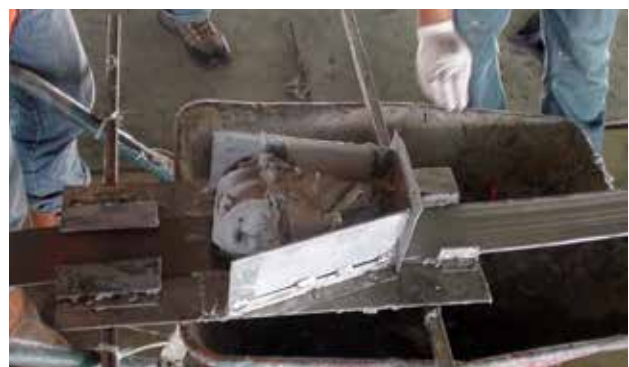
Coating of CarboDur® plates with Sikadur®
