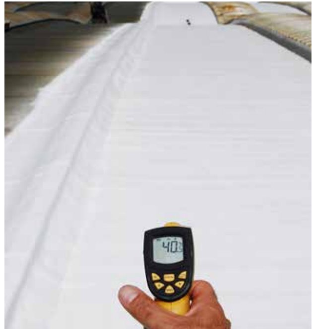
Roof temperature after LAM application.
