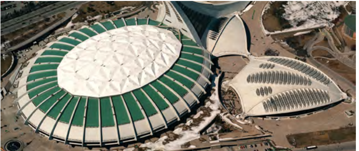
Project year: 2004 | Montreal Olympic Stadium, Montreal, Quebec, Canada Sarnafil® G 410-30, 120 mil membrane webster green
