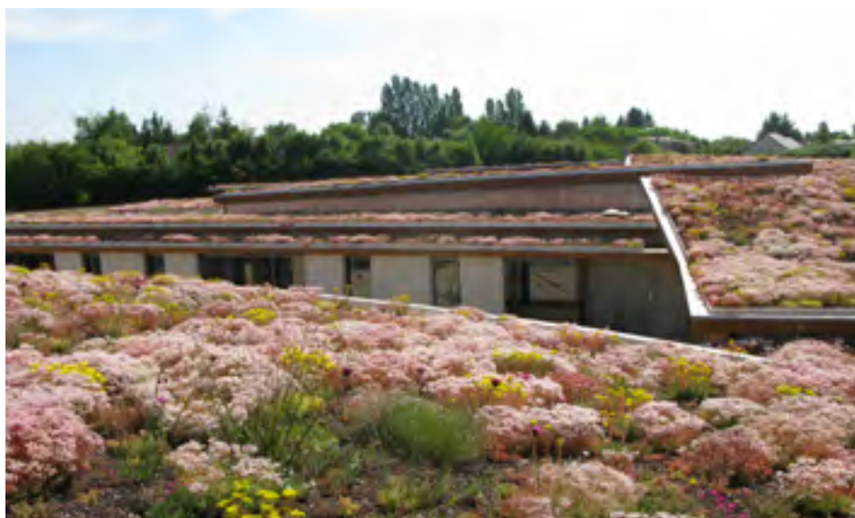
Project year: 2010 | Saint Douillard Medical Center, Cher, France Sarnafil® TG
