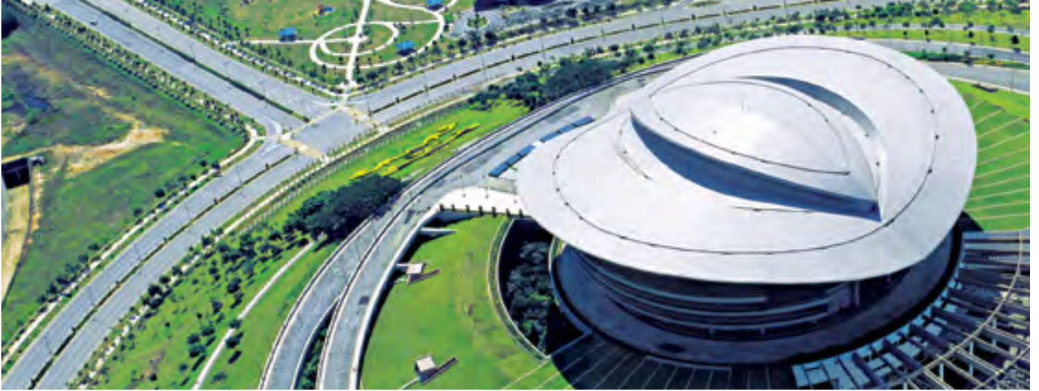
Project year: 2002 | Putrajaya Convention Centre, Putrajaya, Malaysia Sarnafil® S 327-15, Champagne colour
