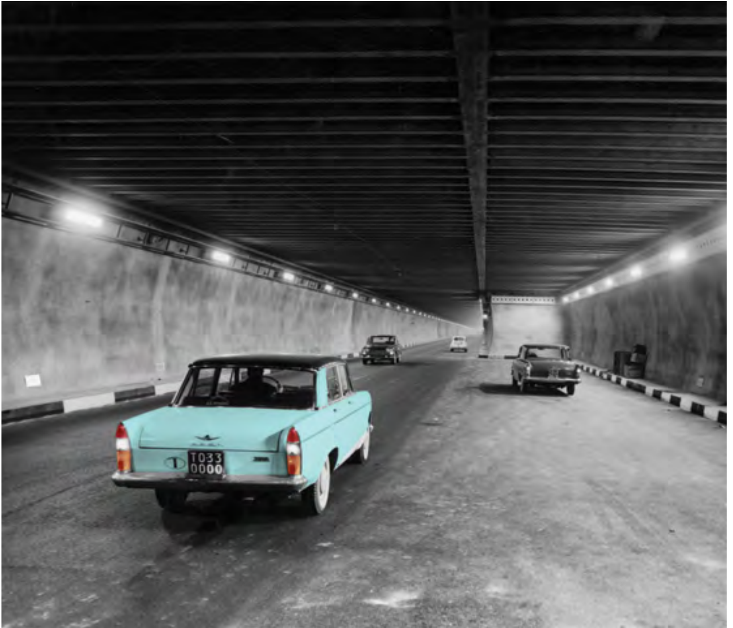
Project year: 1967 | The first tunnel isolation project: Tunnel Gei, Switzerland
