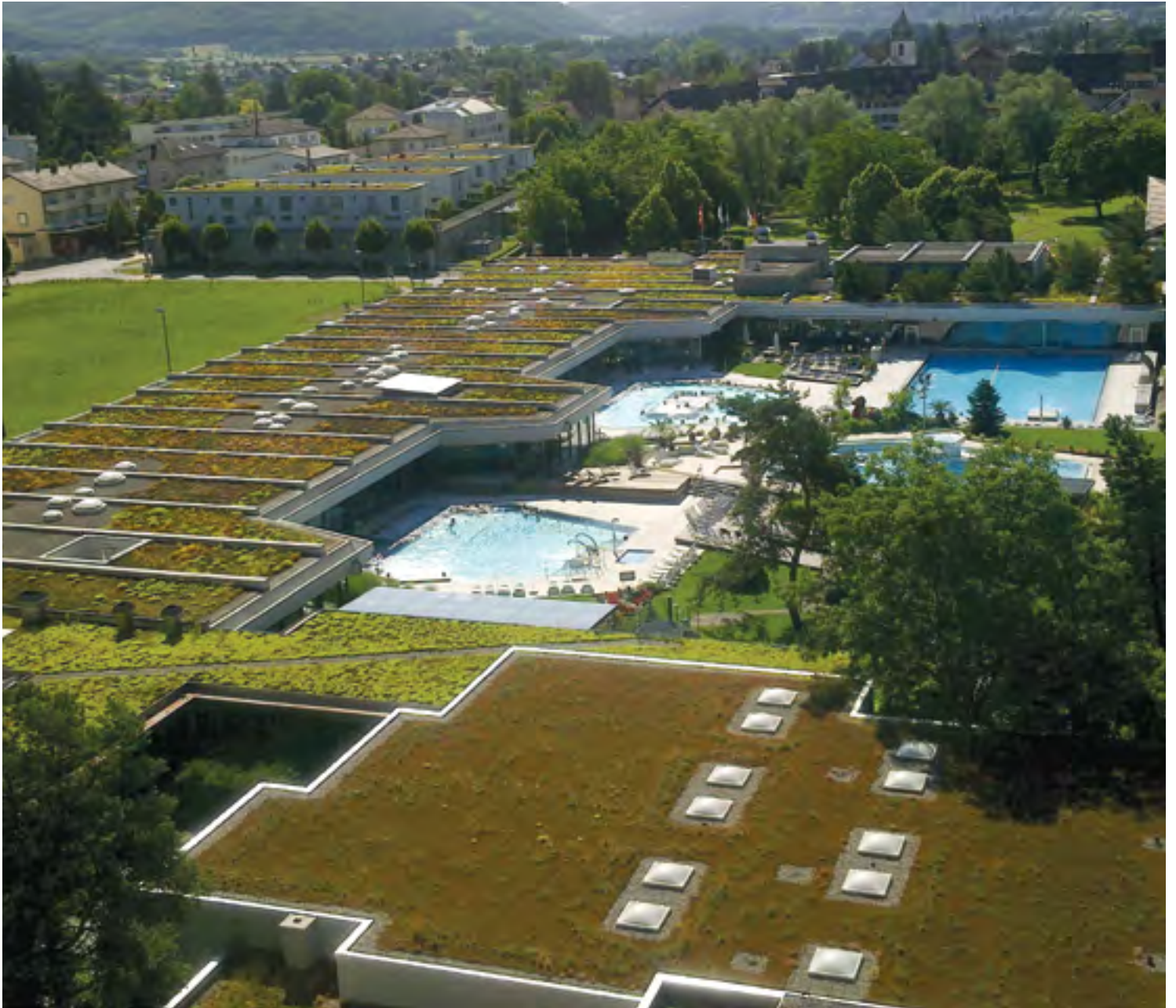
Project year: 1969 | The first project of green roof installation at Thermal Bath, Bad Zurzach, Switzerland
