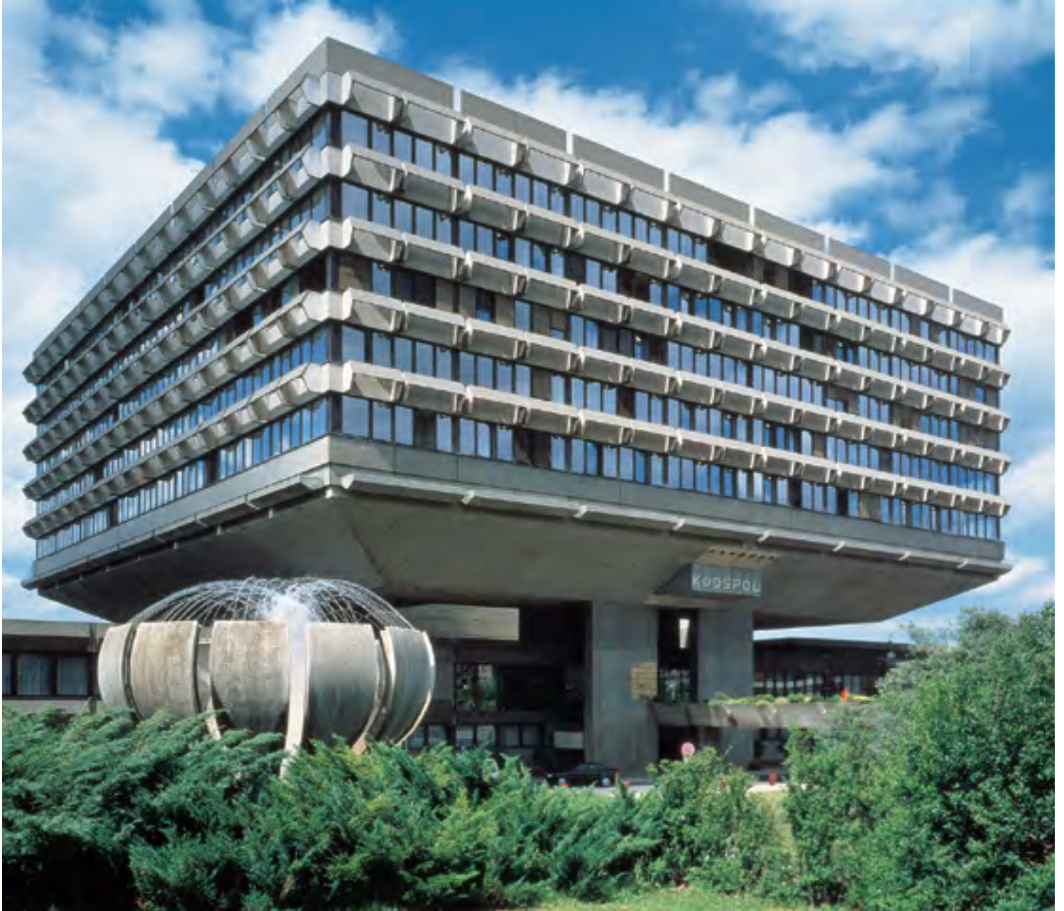
Project year: 1986 | Koospol, Praha 6, Czech Republic Sarnafil® G 441-24E
