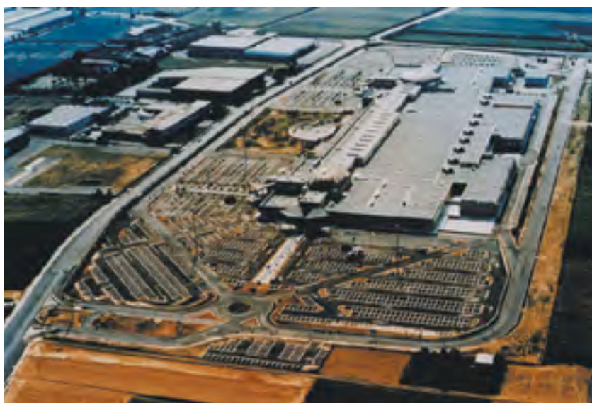
Project year: 1990 | Curno Shopping Center, Curno, Italy Sarnafil® G 442-15; Sarnafil® G 476-15; Sarnafil® G 476-20
