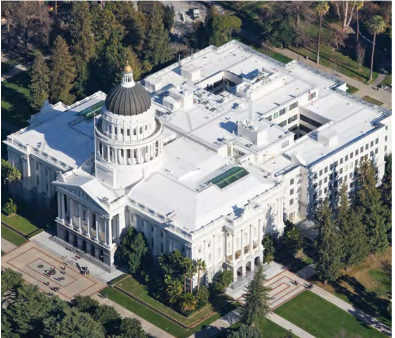
Project year: 2009 | California State House, Sacramento, California, USA Sarnafil® EnergySmart
