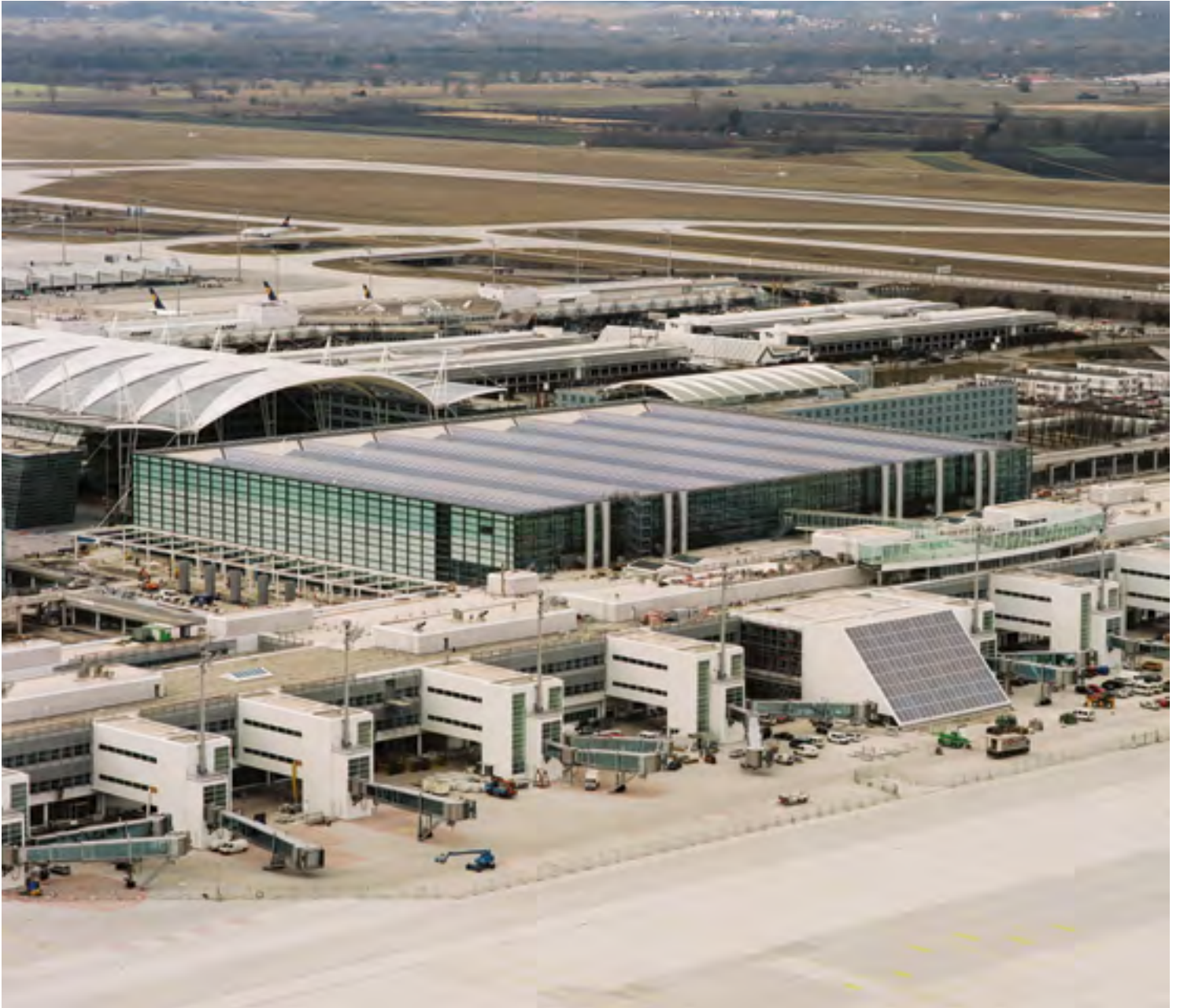
Project year: 1996 | Airport Terminal 2, Munich, Germany
