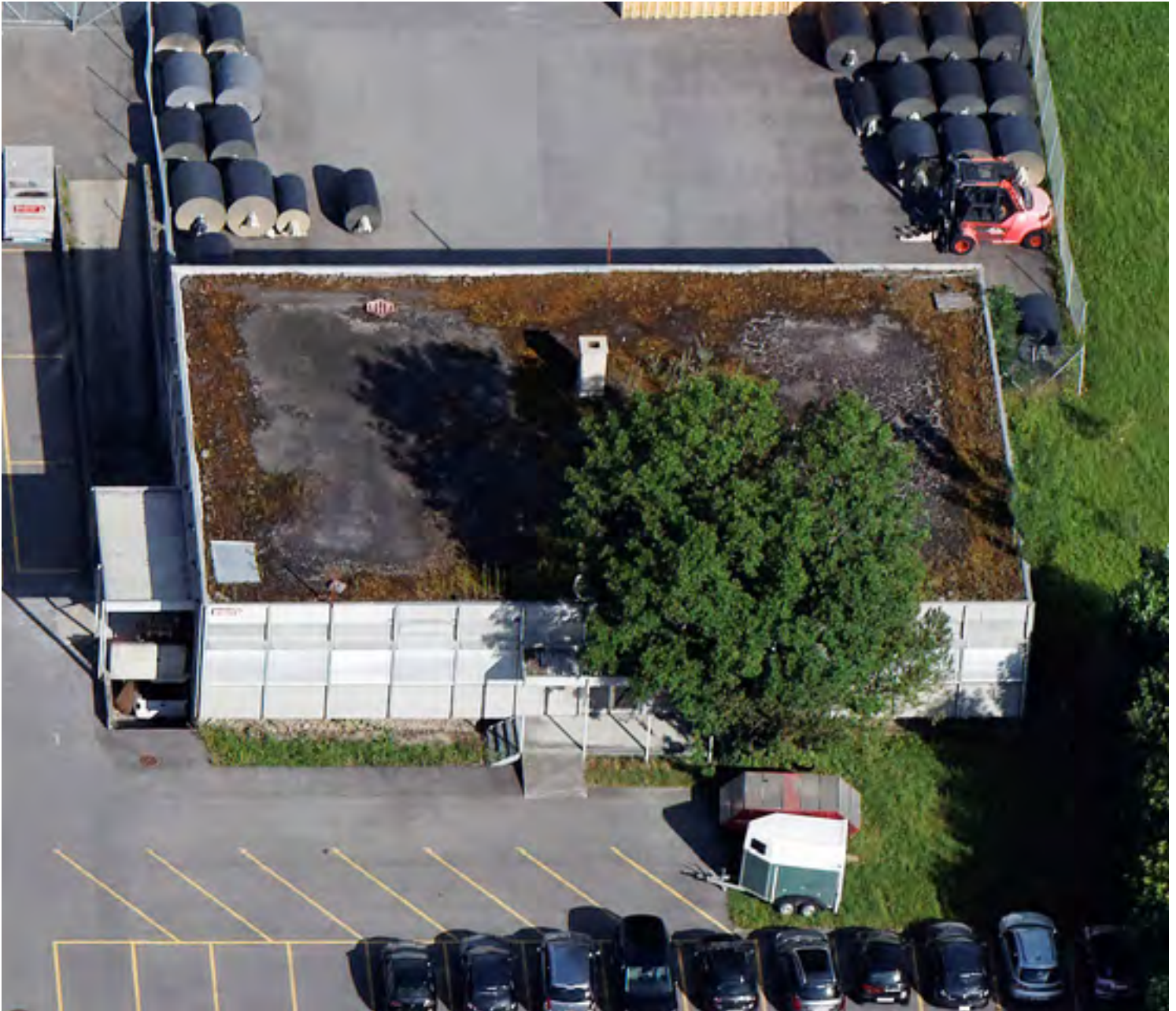
Project year: 1965 | Disa Electro AG, Sarnen, Switzerland Sarnafil® S 21327
