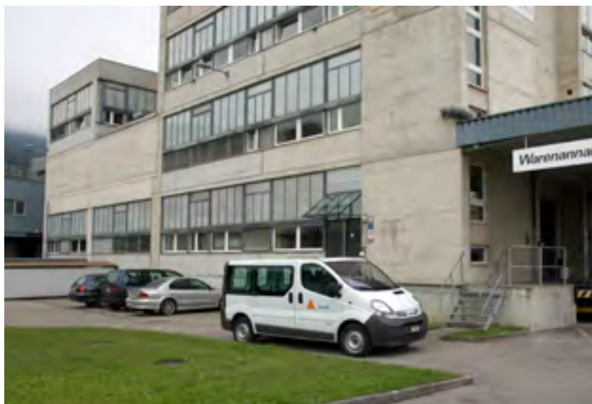
Project year: 1989 | The first Sarnafil® T project at Warehouse Sarnafil, Sarnen, Switzerland
