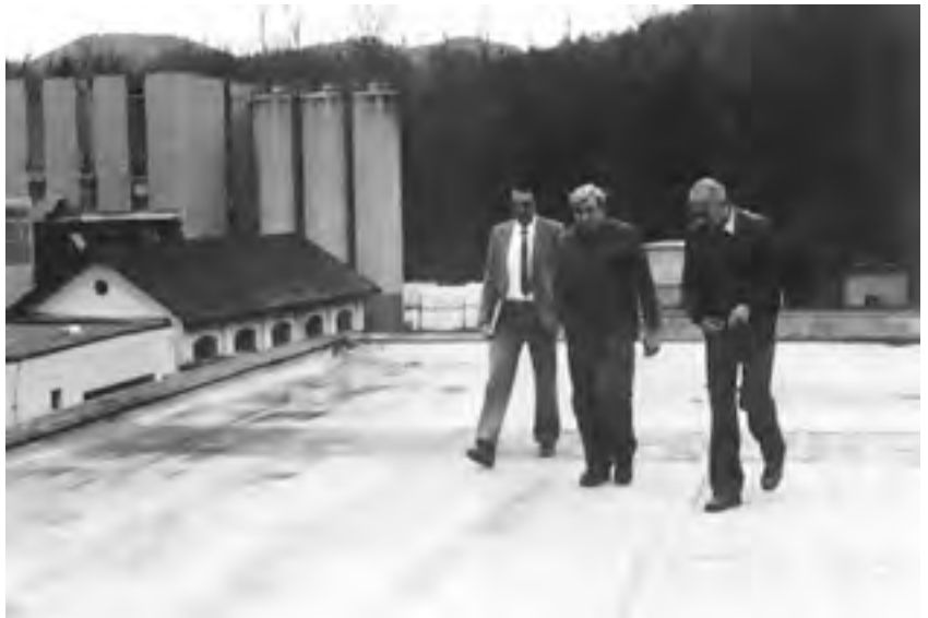
Project year: 1964 | Industrial building of Galban AG, Burgdorf, Switzerland Roof was renovated in 2010
