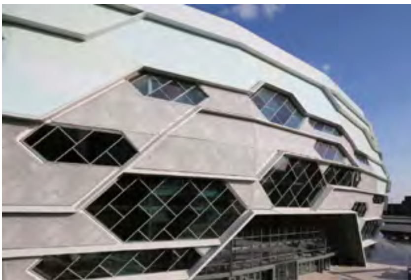
Project year: 2013 | Leeds Arena, UK Sarnafil® S 327-18EL
