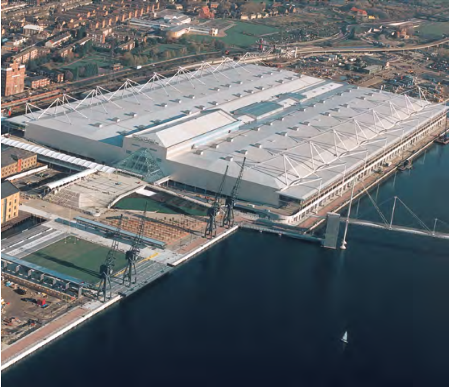
Project year: 2000 | ExCel Exhibition Centre, London, UK Sarnafil® S 327 and walkway plates
