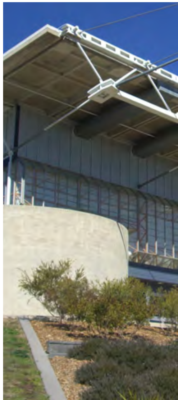
Project year: 1981 | Australian Institute of Sport AIS Arena Canberra, Australia
