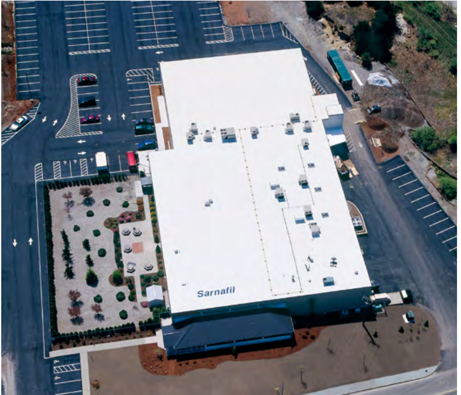
1998 | Introduction of EnergySmart white membrane to reduce building energy consumption due to its high reflectivity of sunlight
