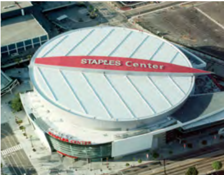
Project year: 1998 | Staples Center, Los Angeles, CA, USA Sarnafil® S 327, Sarnafil® G 410 custom matched "Staples Red" for backdrop of Logo
