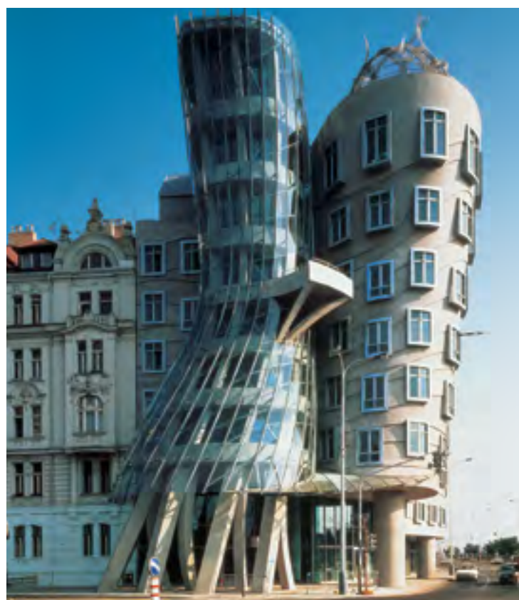
Project year: 1996 | Nationale Nederlanden Building, Praha 2, Czech Republic
