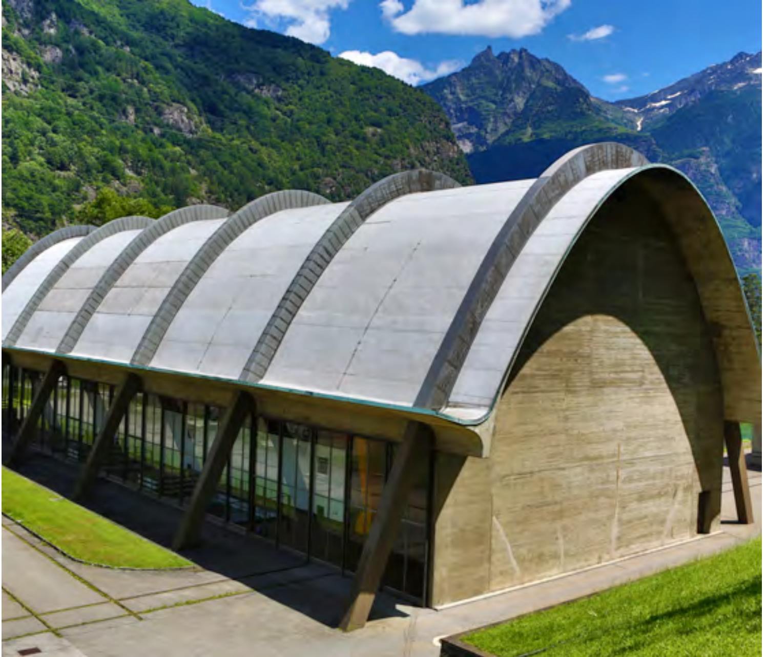
Project year: 1967 | Nuova Biaschina Hydroelectric Plant, Personico, Switzerland | Sarnafil® G 410-12
