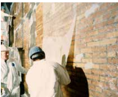
SEISMIC UPGRADING /EARTHQUAKE DAMAGE REPAIR
