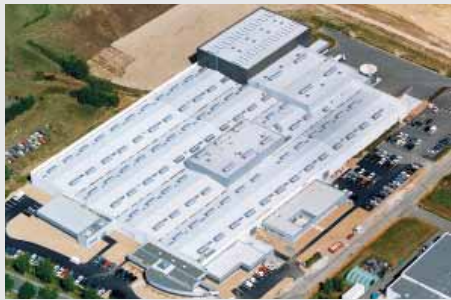
Industrial Building, France
